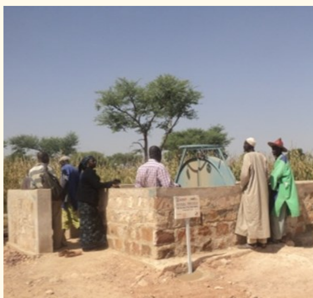
Rehabilitated modern well in Songobia (Bandiagara district)
