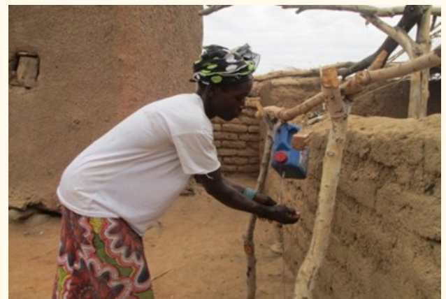
Use of a tippy-tap device installed near the kitchen for handwashing before cooking
